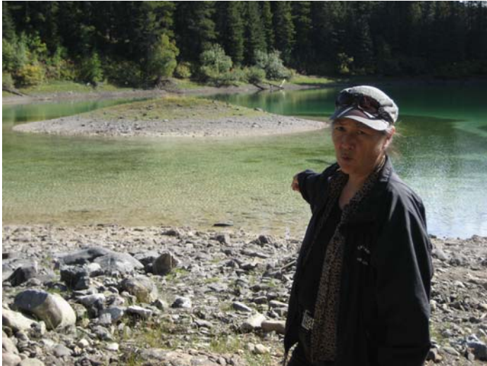
Margo French points to the tailings pond at the abandoned Bralorne-Takla mercury mine. Contamination is evident in the water's color and silt. Use of the water by the nearby Lustdust exploration site has caused the water levels to go down exposing the mound of dirt seen here.
